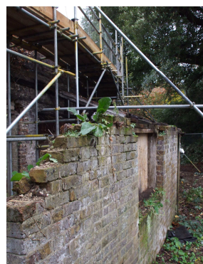
External wall to bothies
